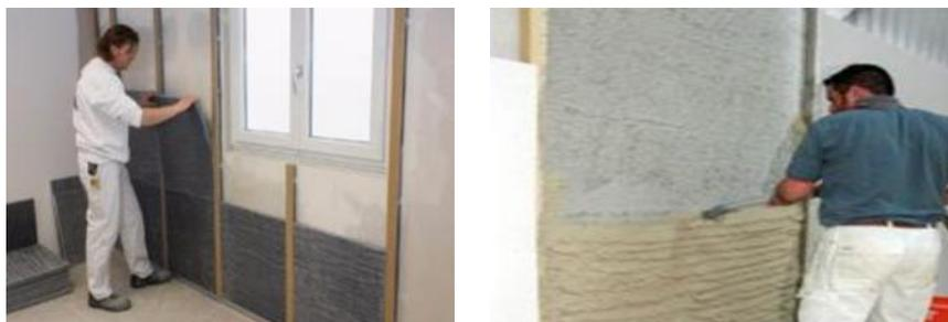
Figur 5. Aerogels application as a thermal insulation for inner wall,
